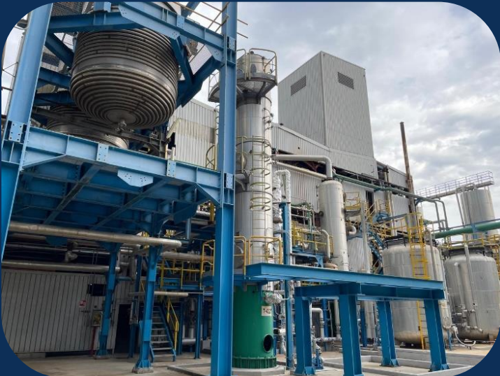
Glycerin distillation column and associated storage and extraction capacity
